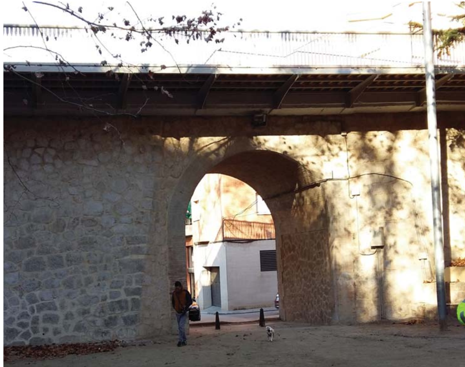
Bridge side view.
