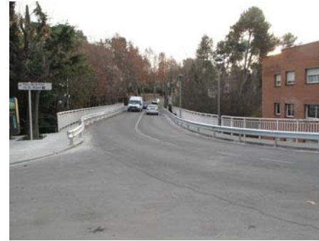
Bridge previous state.
