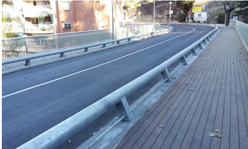
Road and sidewalks on the bridge.
