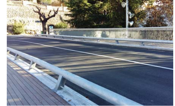
Overpassproof steel curb.
