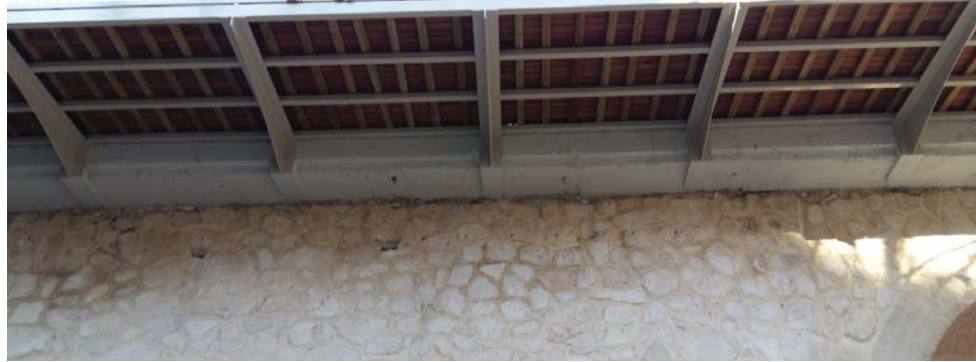
Extension down view.
